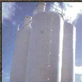
Permanent Storage Tank
